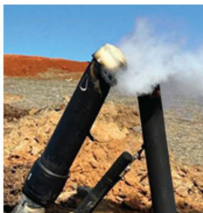
Figure 2 - Subsurface fire due to compromised infrastructure.
